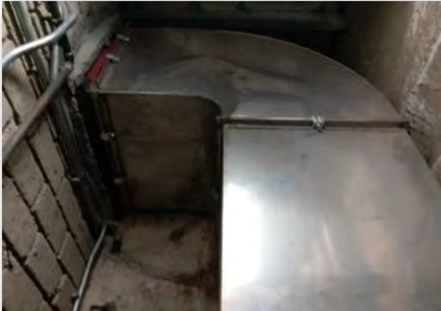
Replacement of New Stainless Steel Air Duct riser for Toilets
